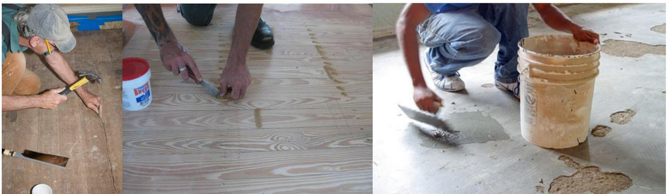
❖ ***Fill any major holes and seal the surface of your floor if you will be applying floor leveller. This should be completed at this stage so you end up with the optimal fresh clean flat and level surface to begin your job.***
